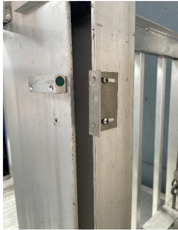
Figure 13. Bracket Installed to the back of the travel beam
